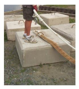
Place the top of the sacrificial end with the swivel through the eye splice on the other side of the mooring ring, as in the following picture.
